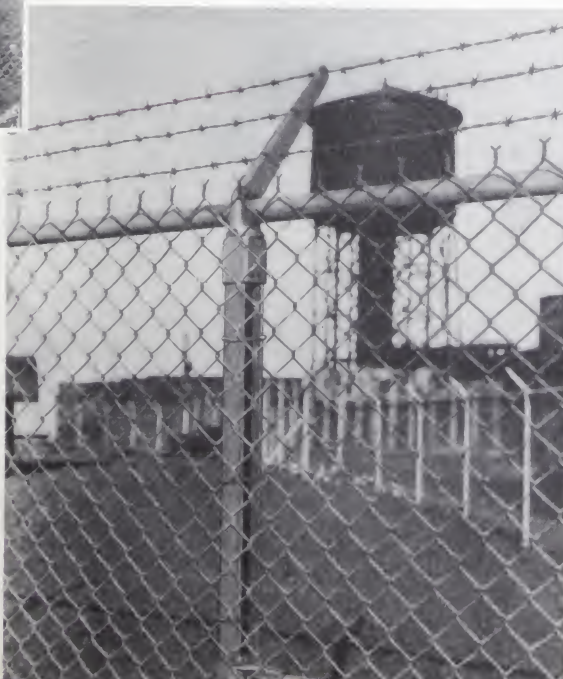
Above is a Cyclone Invincible Fence surrounding a parking yard. The name INVINCIBLE is clearly understood by a glance at the top of it . . . the arms along which barb-wire is strung. This fence is clearly impassable by any ordinary means and is largely used to enclose factory yards and industrial plants generally.
